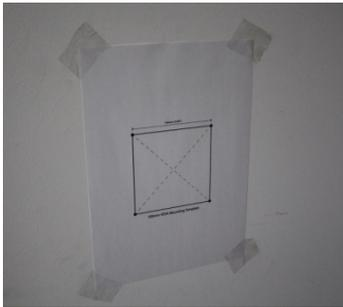
1) Mount provided VESA template to surface and in ideal location. This is often behind and above screen walling mounting brackets, in order that the player is hidden from sight once the screen is in place
